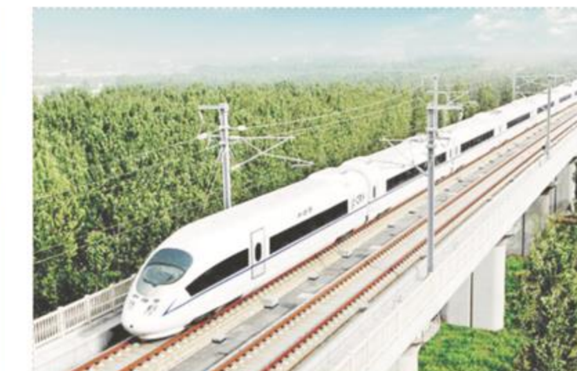
石武高铁 Shi Wu High Speed Rail
