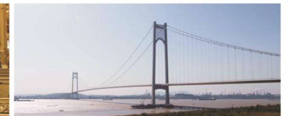
桥梁建设 Bridge Building
